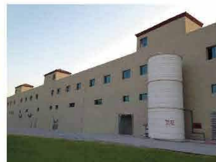
Randhal Project-United Arab Emirates
